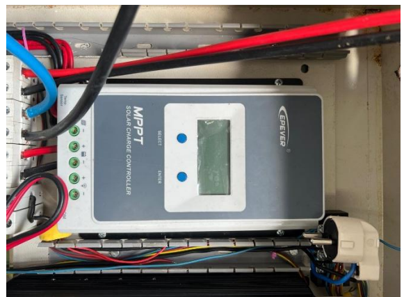
Gambar 12. Solar Charge Controller
