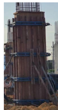
Gambar 2. Bekisting Kolom Semi-Sistem
