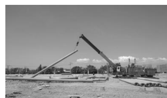
Gambar 4. Liftingpile
